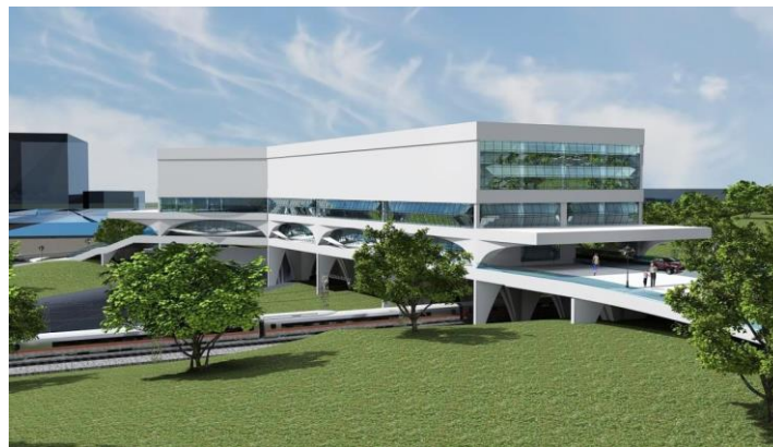
Figure 13. A bridge building with a transport interchange over the connection of two branches of the railroad and the Varshavskoye highway
