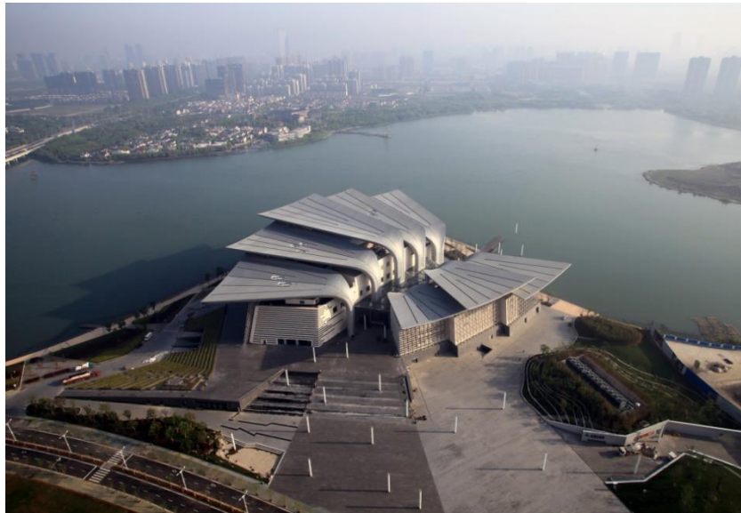
Figure 14. Wuxi Grand Theatre. China. Architecture studio PTS Architects.
