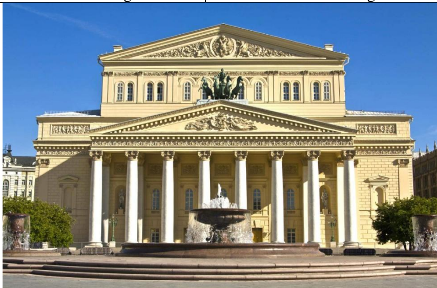
Figure 1c. The main facade of the Bolshoi Opera and Ballet Theatre in Moscow. Historic stage
