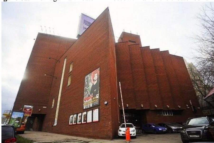
Figure 6b. The Taganka Theater in Moscow. The new part of the theater building
